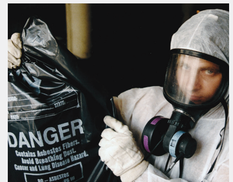
Asbestos Tearout Worker
